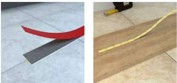
Peel back the film from the adhesive backing Apply directly to a clean surface. The VHB will 'set' within 72 hours for secure fitting.
